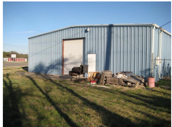
Photo 6 View of light industrial facility west of the site
